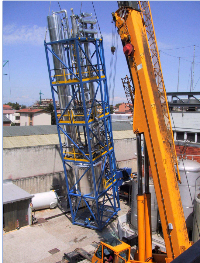
Distillation unit under erection
