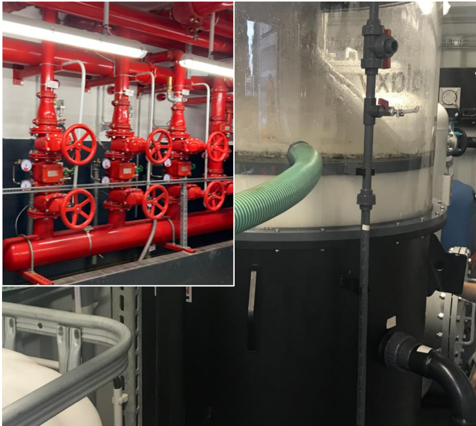
Sprinkler system - foam fractionation unit
